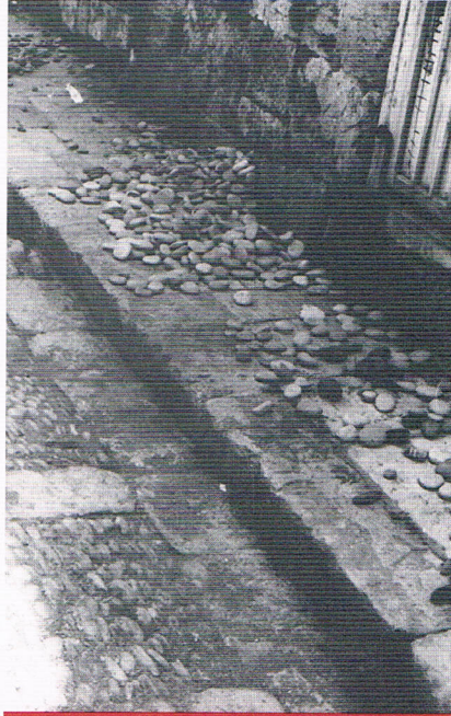
Shingles used as pavement material
