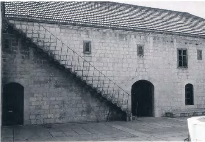
13 Central courtyard, south view. Stone stairway incorporated in the courtyard's south wall leading up to the roof.
